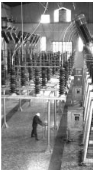
Sala alta tensione (1960) High-tension room (1960)
